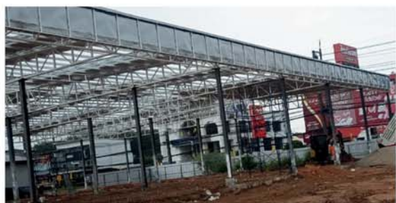
Construction in Progress –Thalang, Phuket
